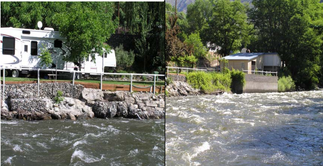
Figure 2. Existing bank stabilization on the west bank.
