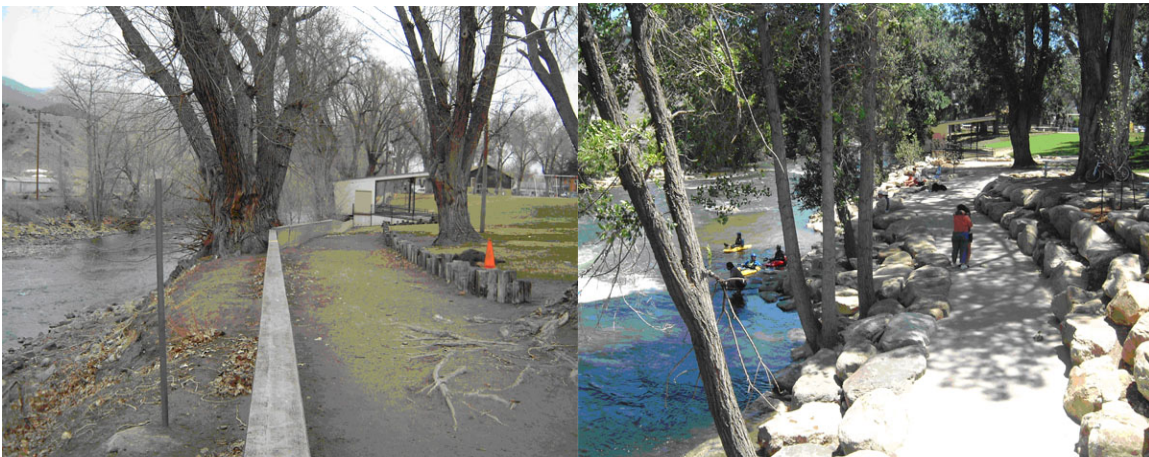
Figure 9. Before and after example of bank terracing and trail
